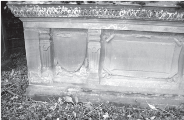
Provost Thomas Bell's Grecian temple with clear signs of lamination.
