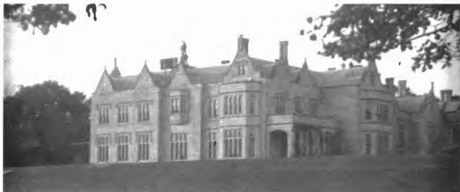
Lisnavagh House, County Carlow
