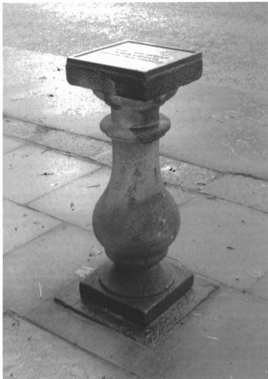
Baluster from Rennie's Waterloo Bridge, London (1817 – 1934) at the Rennie Memorial, Phantassie
